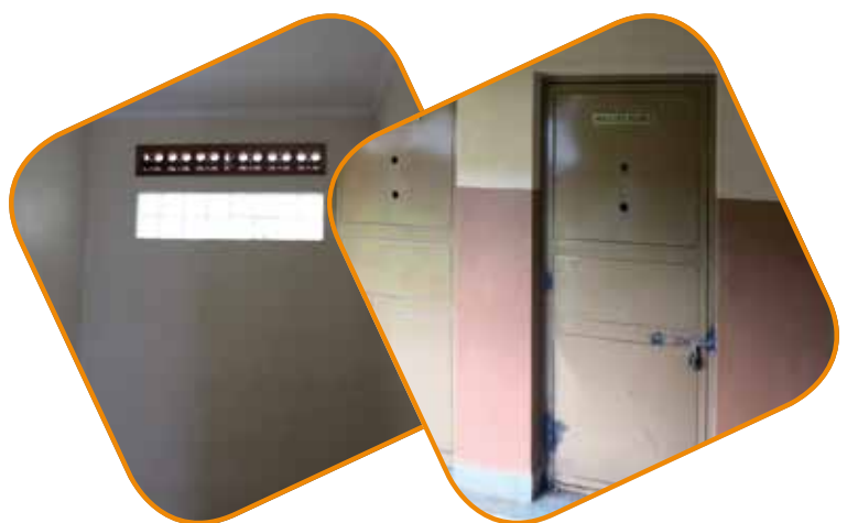
Photos: Seclusion room at Mbale hospital on the left and Mbarara hospital on the right, April 2014. © MDAC.
